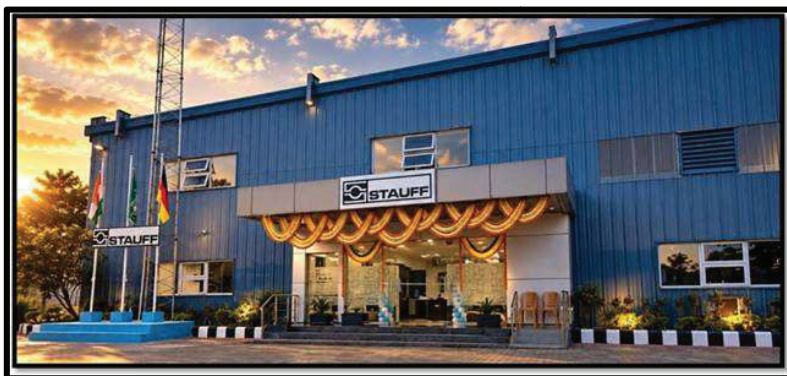
STAUFF INDIA PVT. LTD SEZ UNIT BELGAVI KARNATAKA
