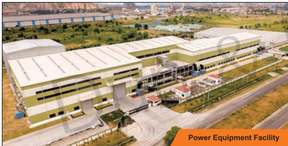
Power Equipment Facility
